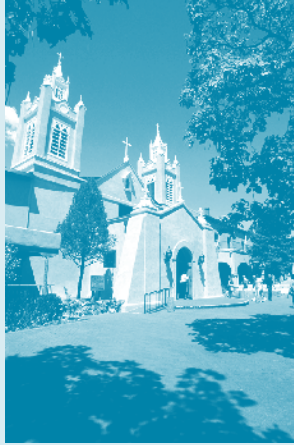
San Felipe de Neri church still stands on the original site in Old Town
